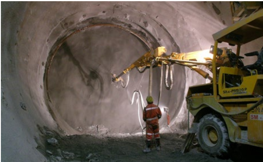
Fig. 2.2: Excavation stabilization with shotcrete
