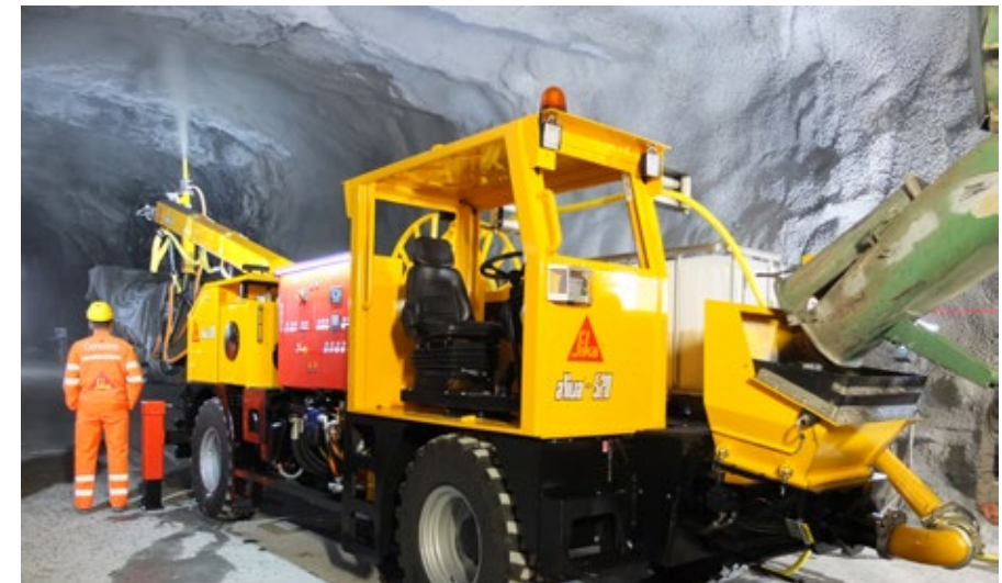
Fig 1.3: Shotcrete application, high degree of mechanization
